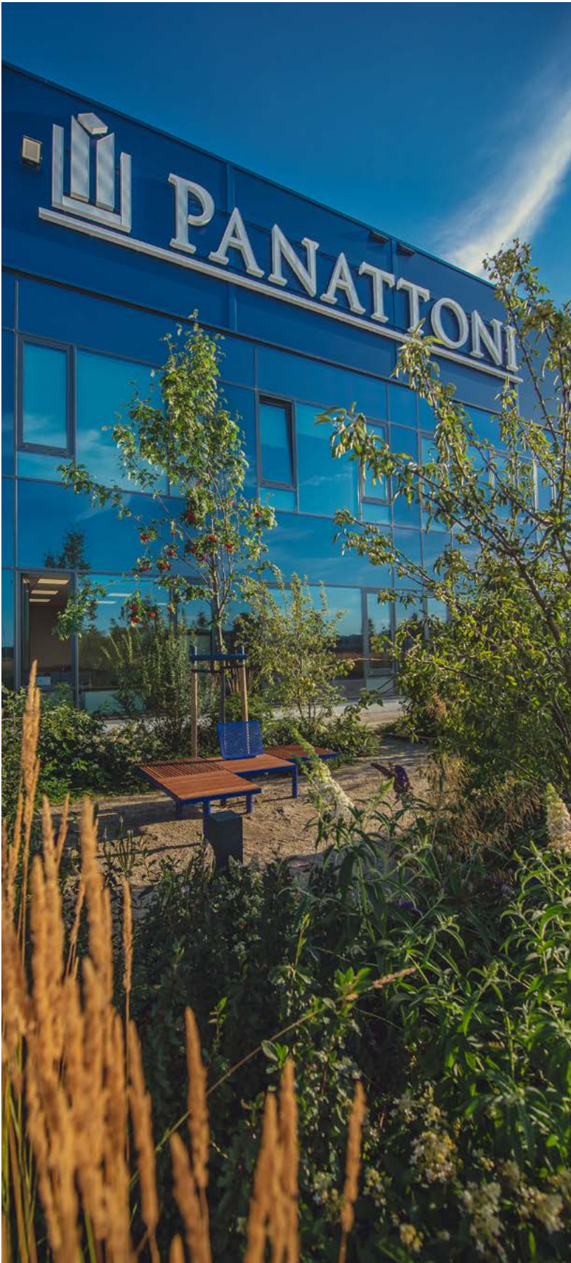
Panattoni Park A2 Warsaw East
