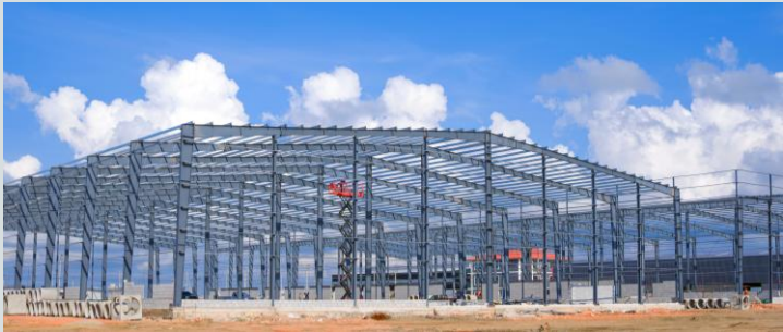
Land Acquisition and a Built-to-Suit Automotive Component Manufacturing Facility in India
