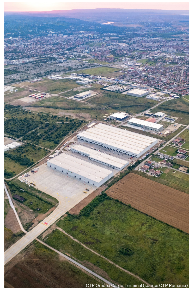
CTP Oradea Cargo Terminal (source CTP Romania)
