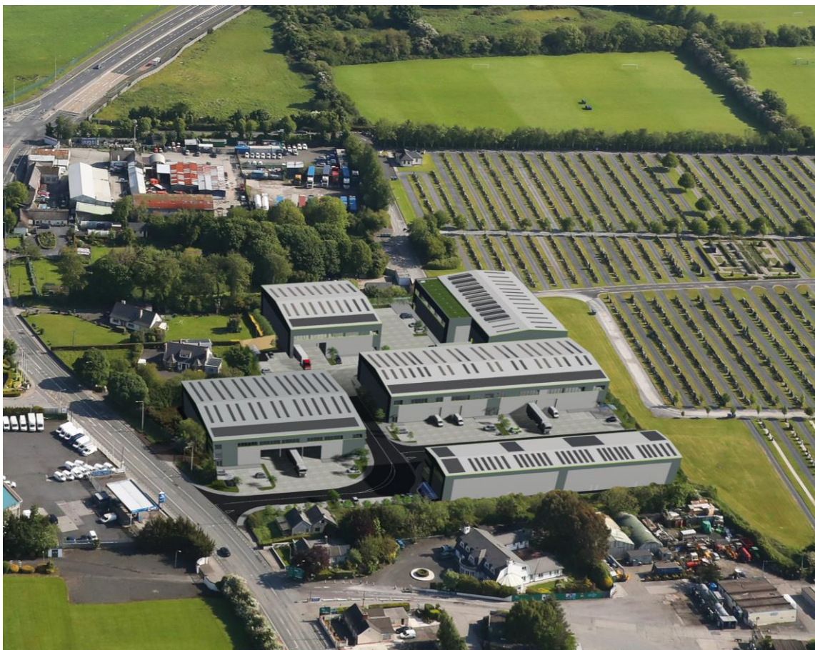
Figure 12: Airport Trade Park; 13 Units Set to Reach Practical Completion in 2026
