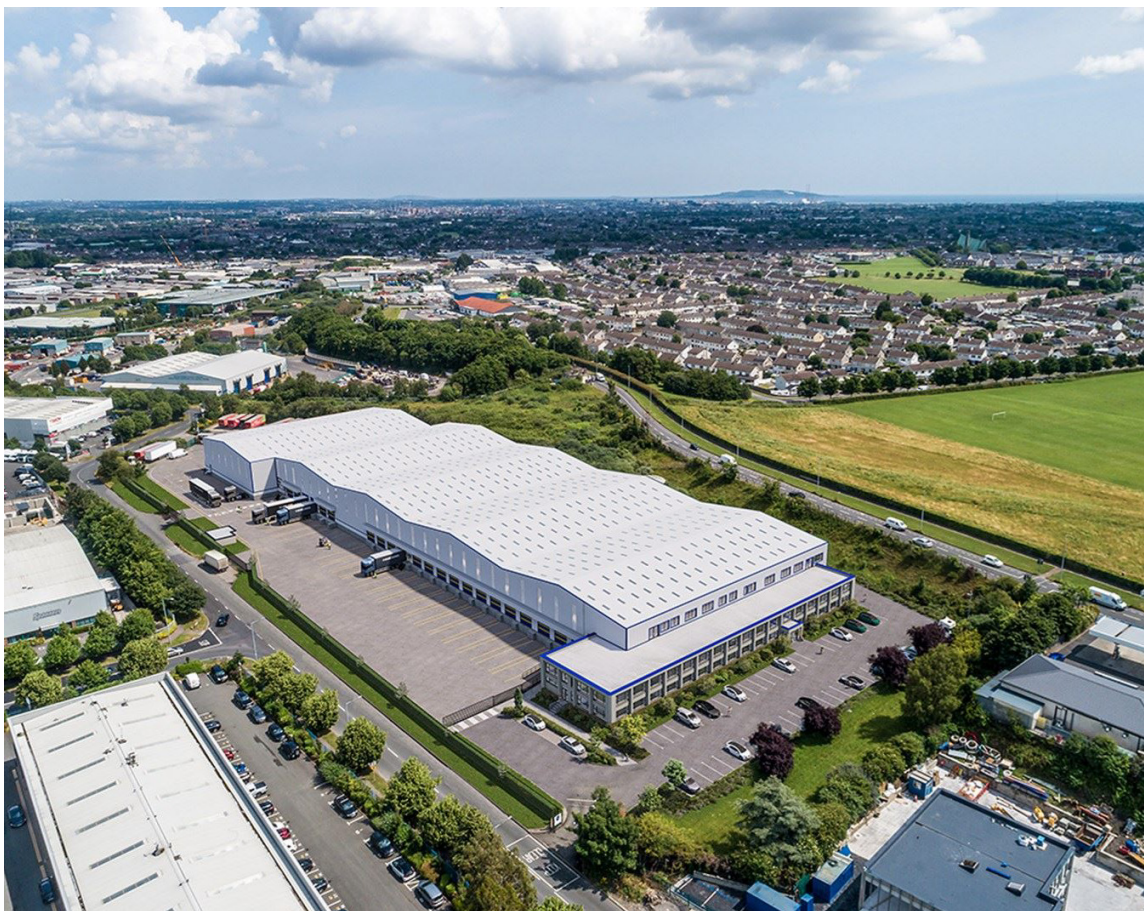
Figure 14: Ballymount Logistics Hub; Refurbished (BER A) and Available From September 2024
