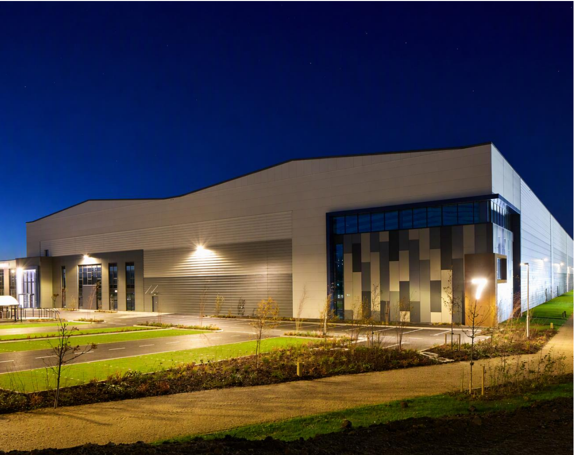
Figure 9: Unit 7, Mountpark Grange Castle West; Let to CEL Critical Power in Q2
