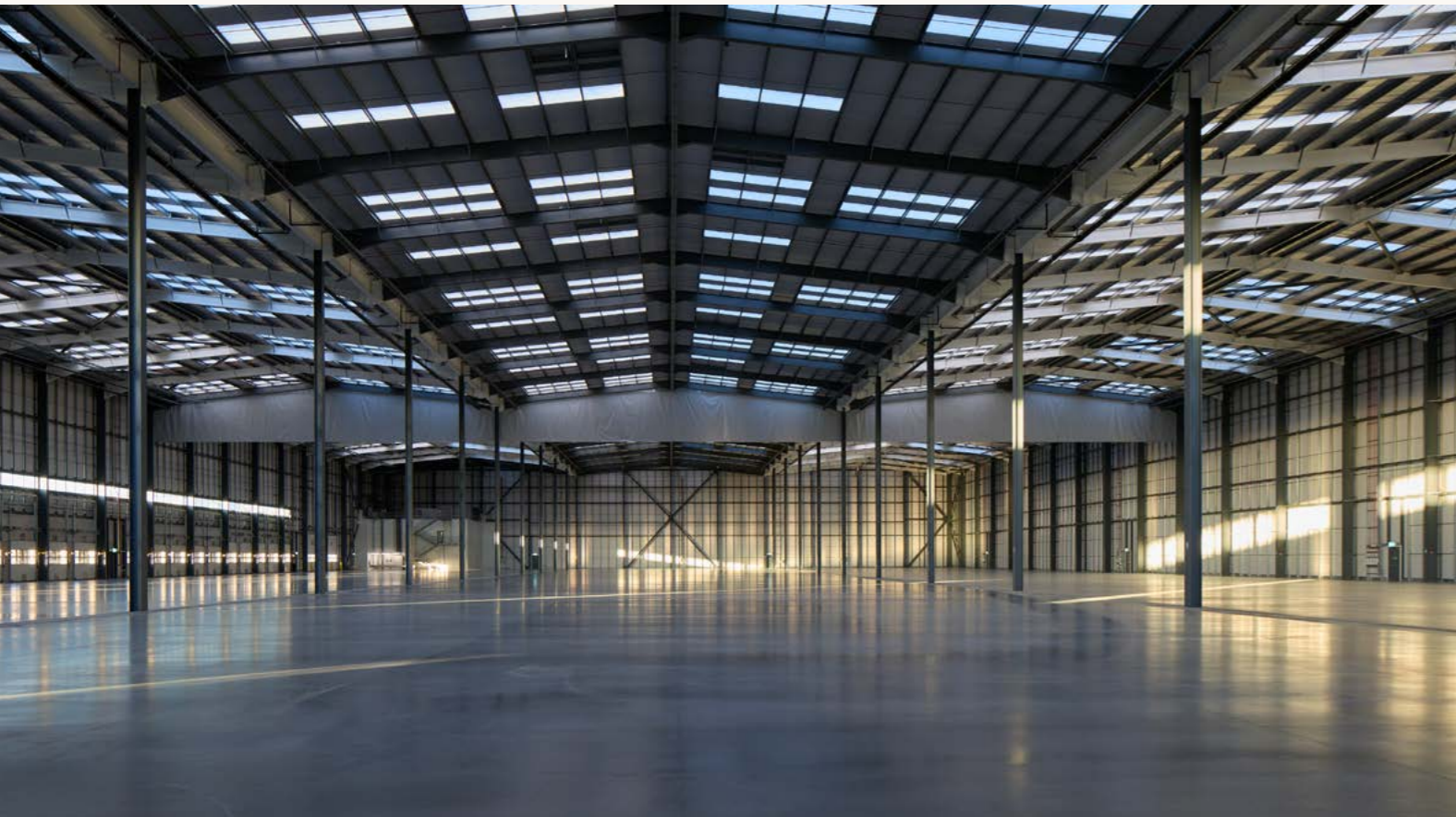
Unit 1 Mountpark Grange Castle West - Mountpark
