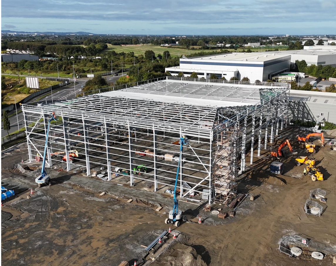
Figure 13: Stadium Business Park, Dublin 15: New Units Under Construction & Available to Let
